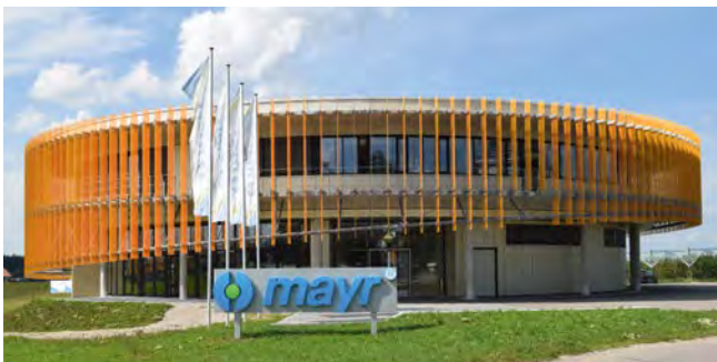
Communications centre mayr.com – Opened 2018.
