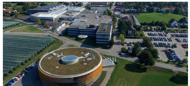
mayr ® headquarters in Mauerstetten
